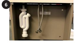
Connect your basin to the drain and the basin tap to your hot/  $\operatorname{\mathsf{cold}}$ connection, it is easy to access the unit from the front to complete this step. please note that this can be time consuming given the small  $% \left\{ 1,2,\ldots ,n\right\}$ workspace available.
