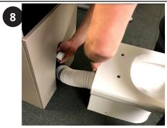
Connect the flush pipe and flexible flush pipe and attach to the pan. You  $\,$ may need to cut down the flushpipe to get the correct fit.
